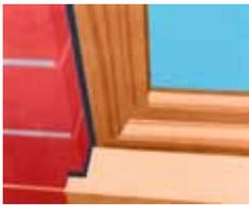
Recommended for the perimeter sealing of timber frames and where overpainting of sealant is required.
